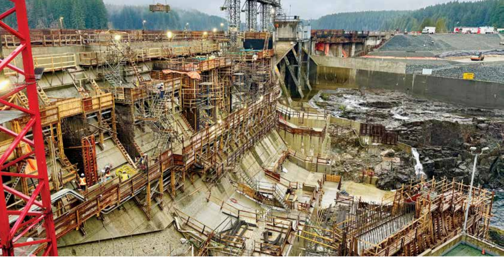
Concrete work on the downstream overflow spillway facility.
