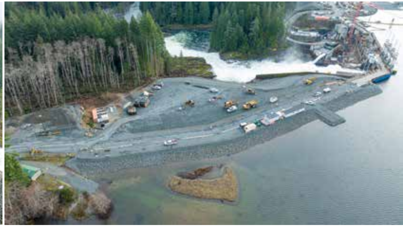
View of the downstream berm work.
