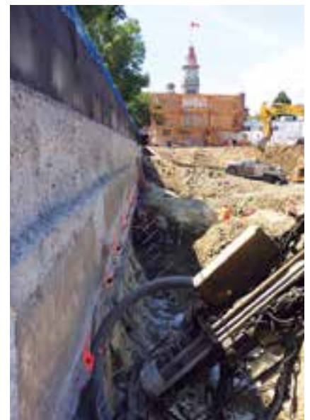
Tie-back drilling works for the shoring operations.
