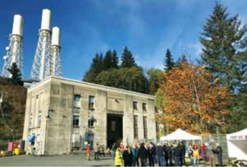
Low-level outlet works just downstream of the John Hart dam.
