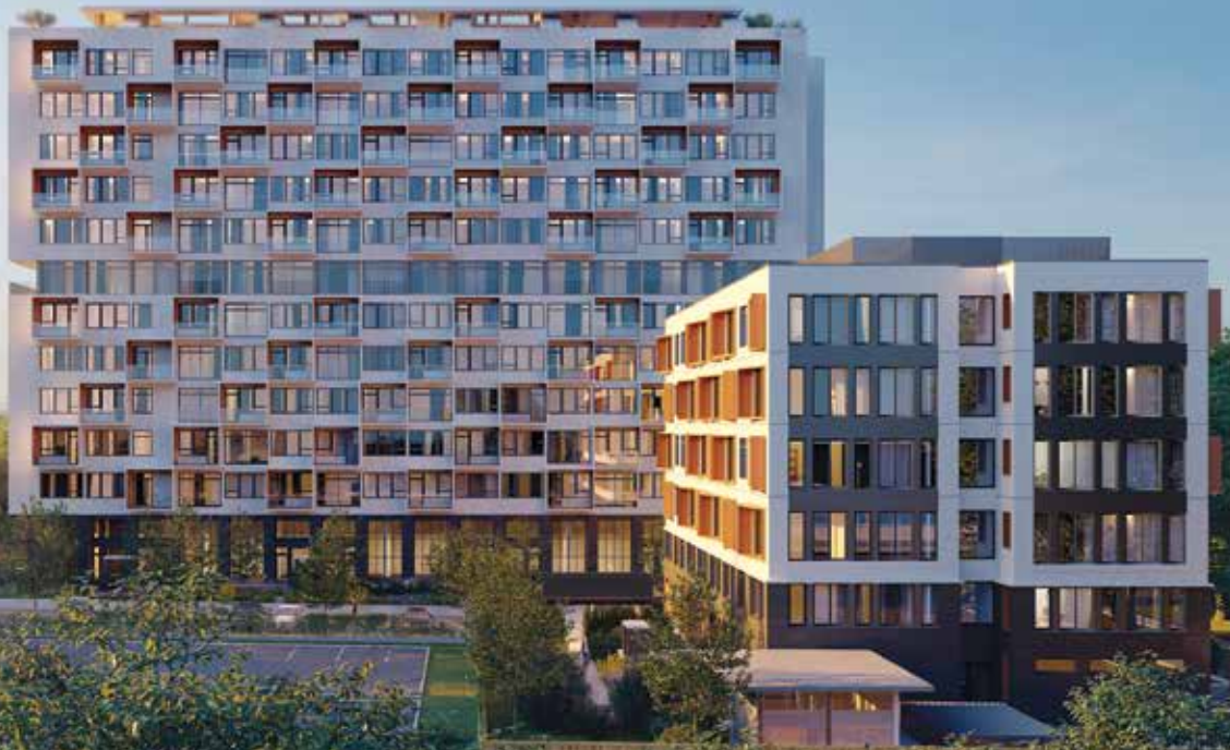
Tresah West, a 12-storey mass-timber residential high-rise offering 179 residences; Tresah East, a six-storey, wood-frame building offering 66 residences.
