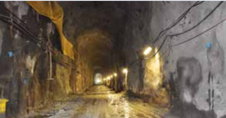
Tailrace tunnel that runs about 600 metres from the powerhouse to the Campbell River.
