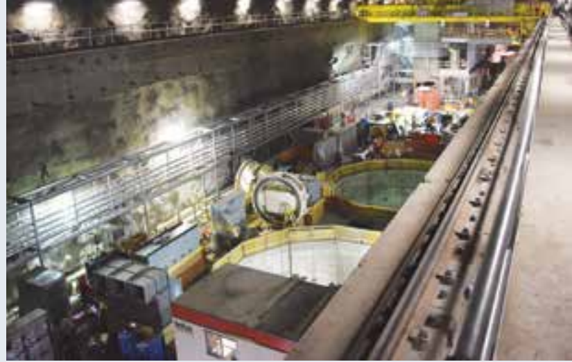
Progress on the underground powerhouse taken December 11, 2017.
