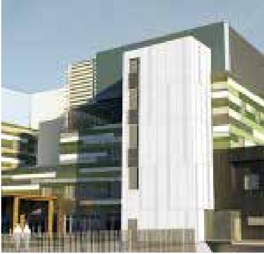
North Island Hospital Comox Valley.
