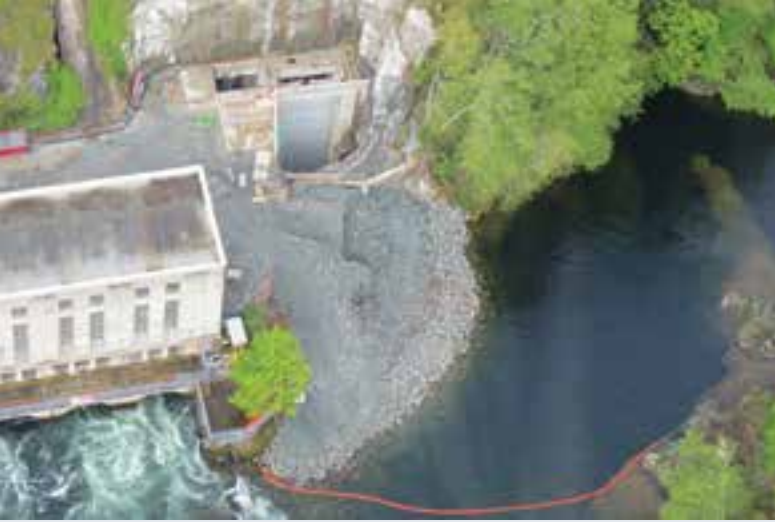
The tailrace tunnel outlet where water from the tunnels will re-enter the Campbell River, near the existing powerhouse that's 70 years old. The rock plug is planned to be removed at the end of 2017.
